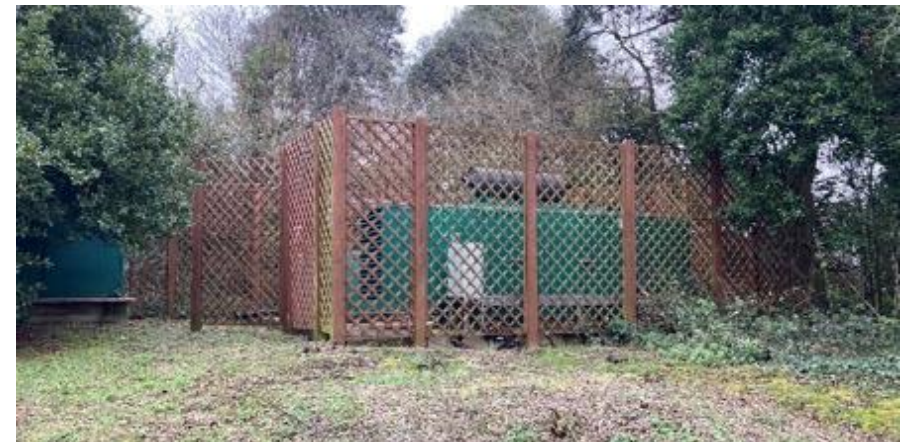
Figure 28: Plant within the grounds of Goring Hall
