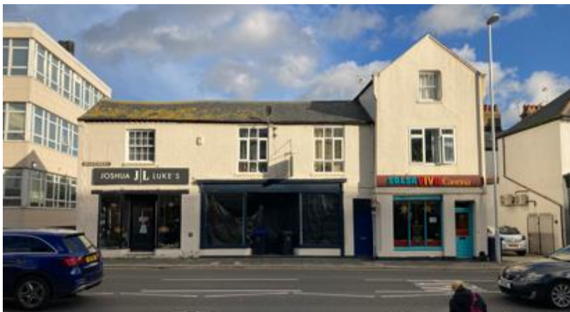
Figure 20: 28, 30 and 30a High Street, formerly cottages associated with Warwick House
