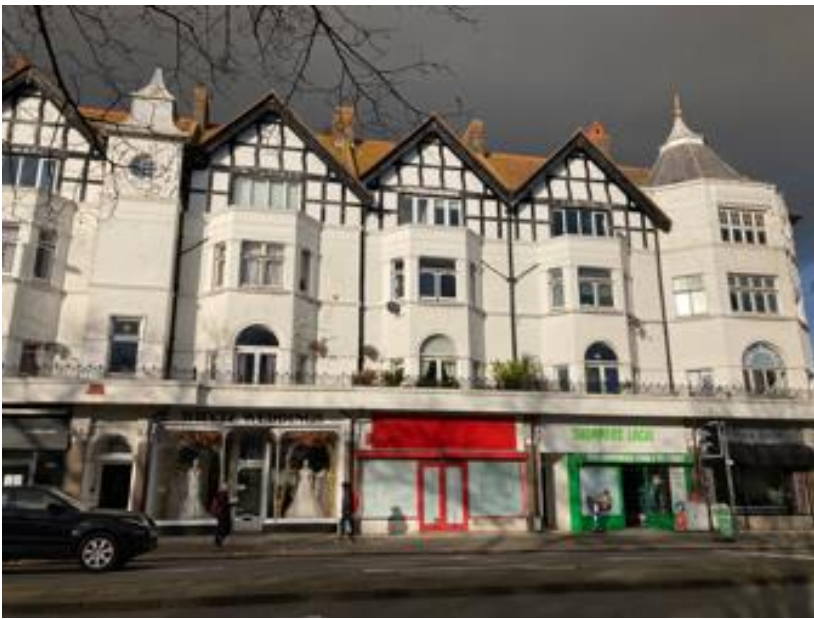
Figure 76: Variable quality shopfronts at Broadway Mansions
