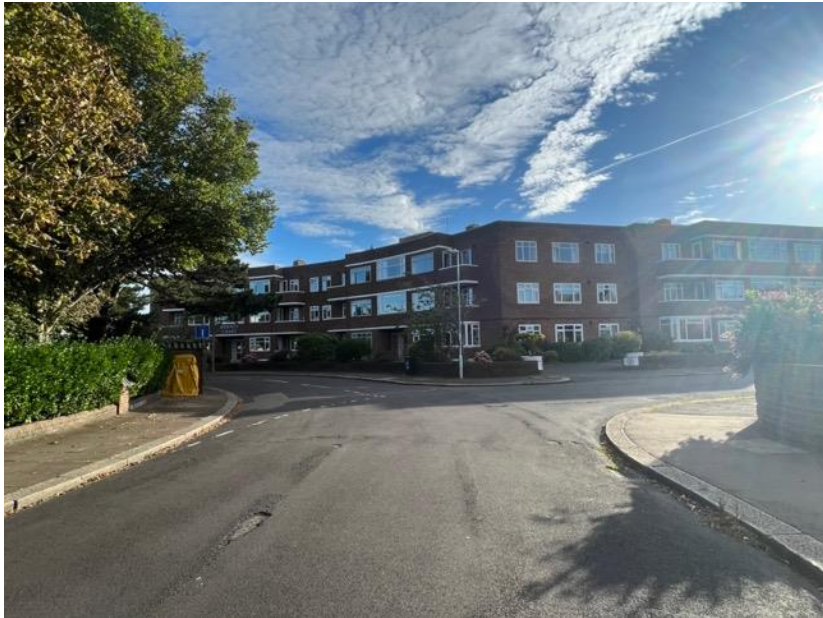
Figure 41: View towards Romney Court from Winchelsea Gardens
