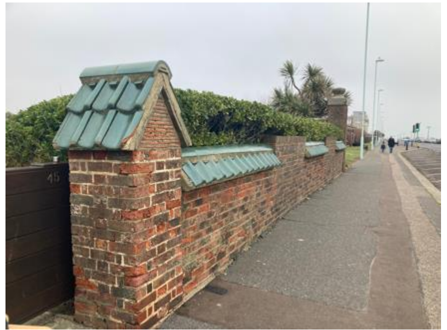
Figure 16: Brick boundary walls with green pantile capping
