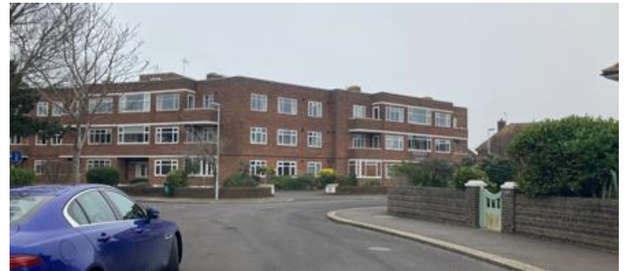
Figure 35: Low brick boundary walls around Winchelsea Gardens
