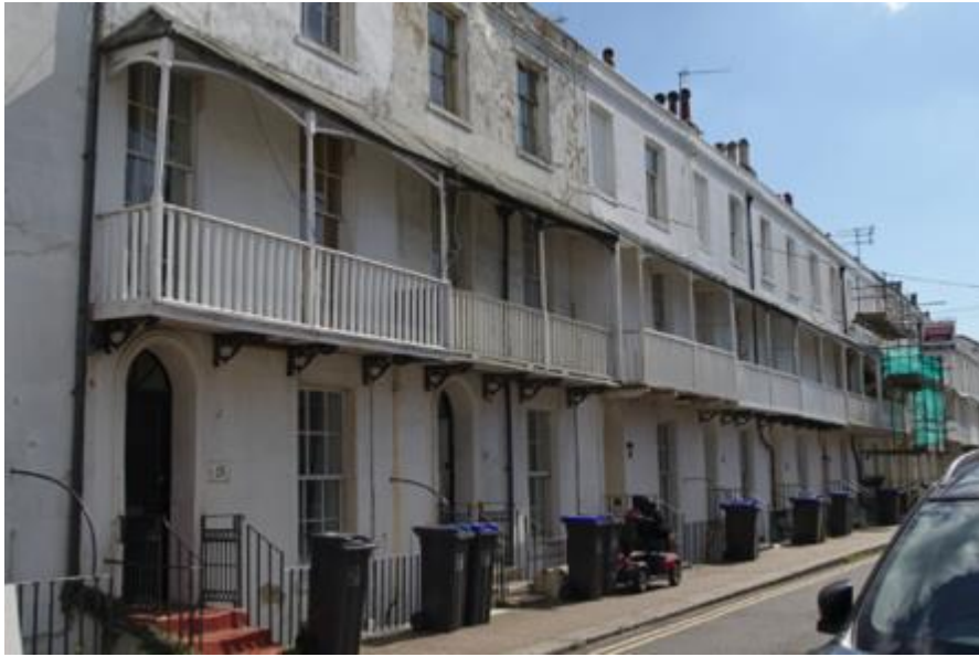
Figure 34: Early 19 th century terrace on Warwick Road
