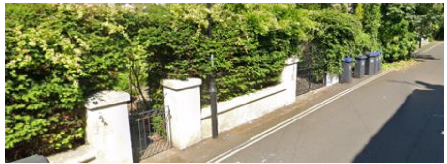
Figure 54: West side of Warwick Place
