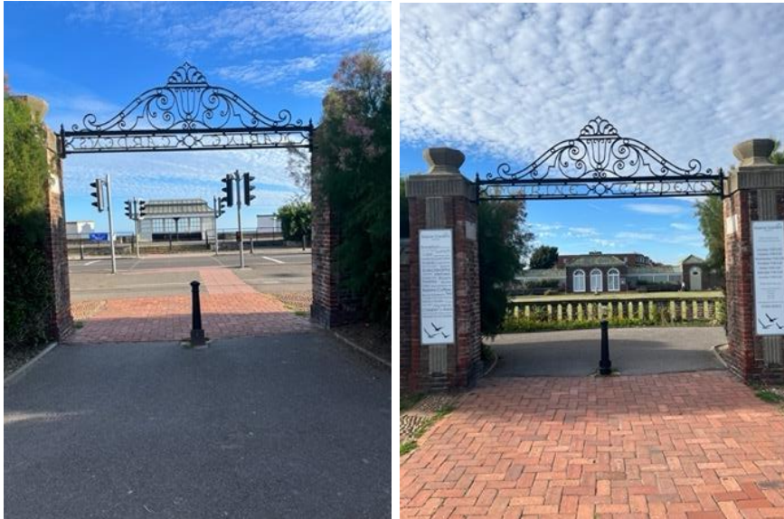
Figure 36: View north and south from entrance gates
