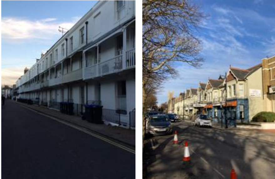
Figure 13: Examples of residential buildings on Warwick Road (left) and Steyne Gardens (right)
