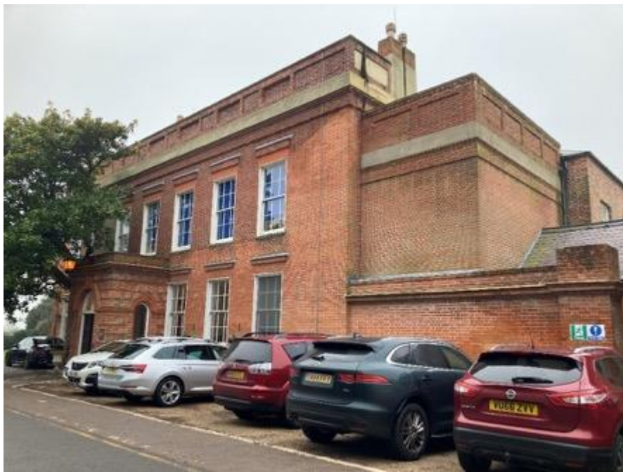
Figure 20: East facing elevation of Goring Hall with parking to front
