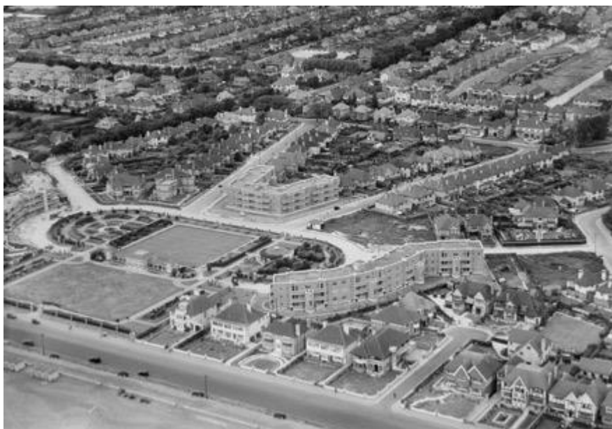
Figure 12: Marine Gardens, view from the south; 1937; Source: Historic England
