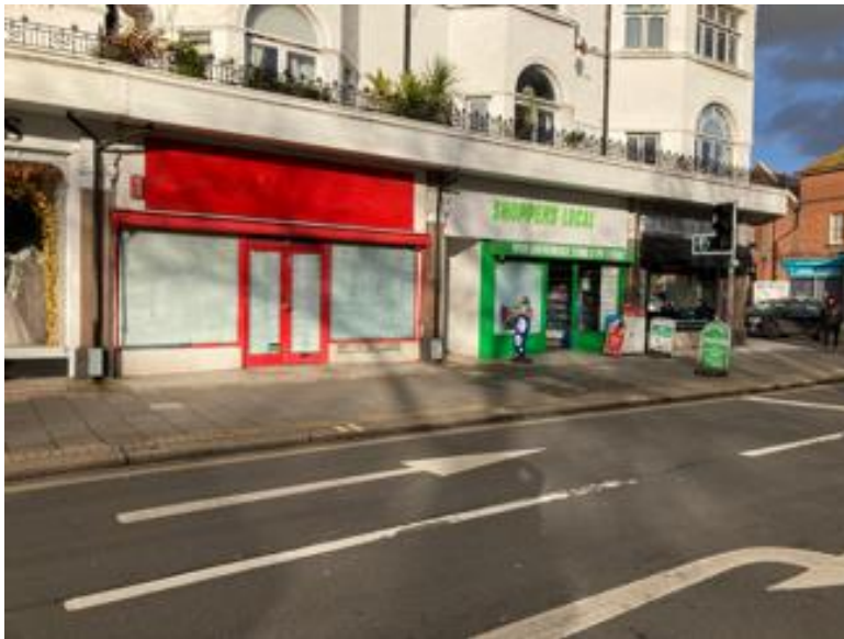
Figure 61: Poor quality shop fronts along Brighton Road
