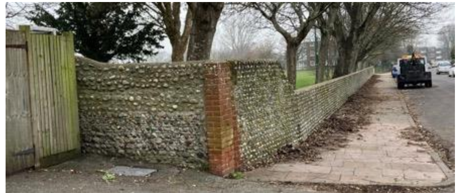
Figure 17: Flint wall to the north of The Bull's Head within the conservation area.
