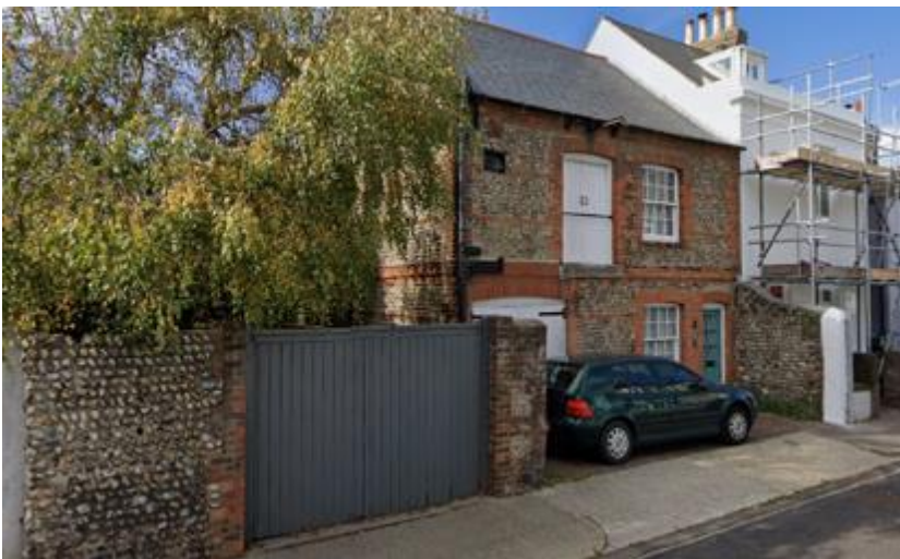
Figure 48: Park Road, west side
